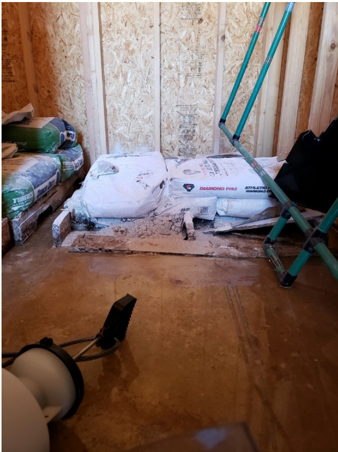
Photo: Standing water in the equipment shed
