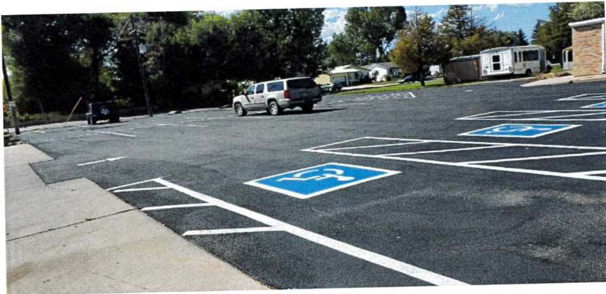
Example of seal coat/ crack fill project
