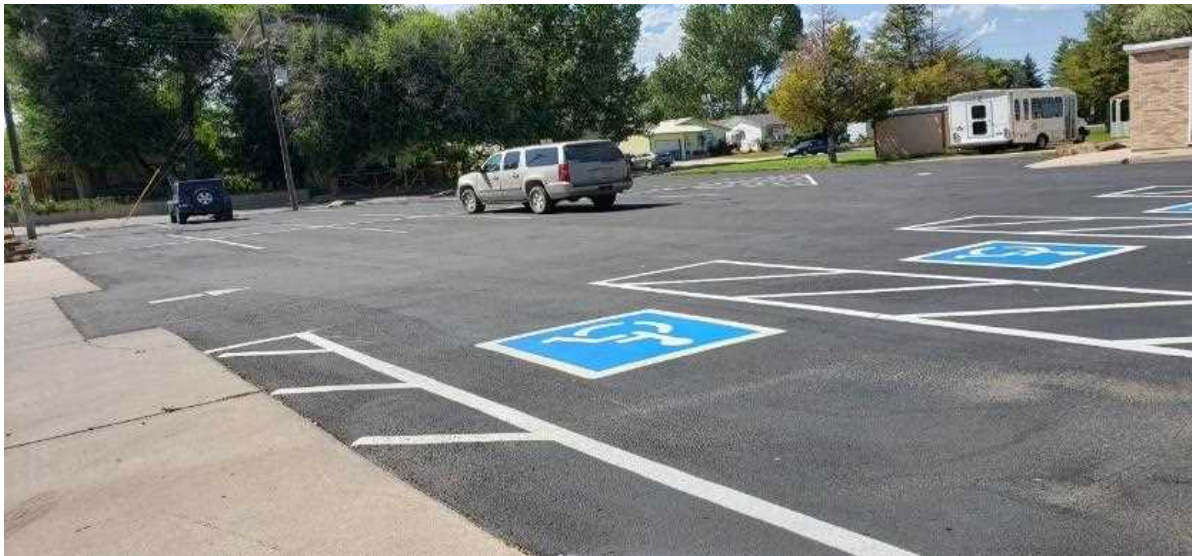
Example of seal coat/ crack fill project
