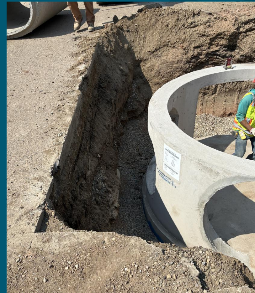
Aesbestos (abandoned) waterline required removal by hazardous waste abatement.
