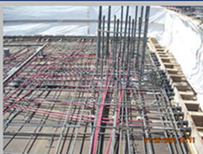
Post Tension Slab Project
