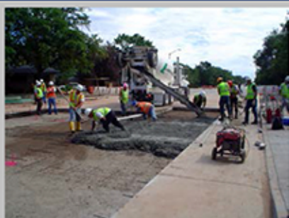
Concrete Paving Project
