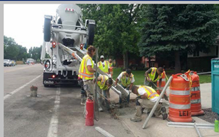
Municipal Concrete – Curb & Sidewalk
