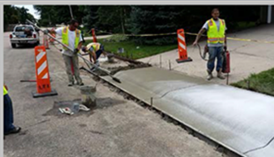
Municipal – Curb & Gutter Project
