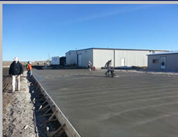
Commercial Concrete – Finishing
