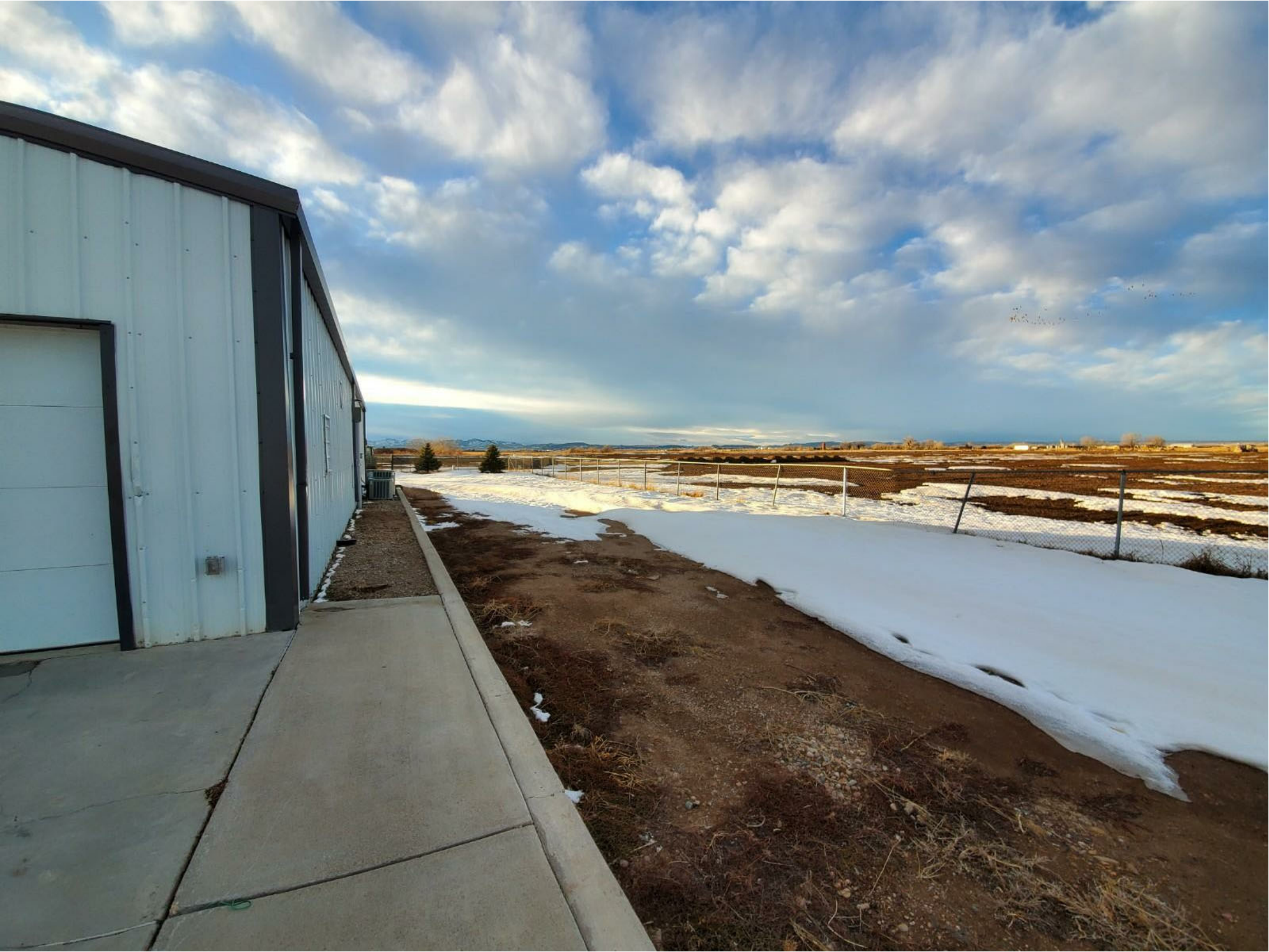
NE CORNER LOOKING WEST
