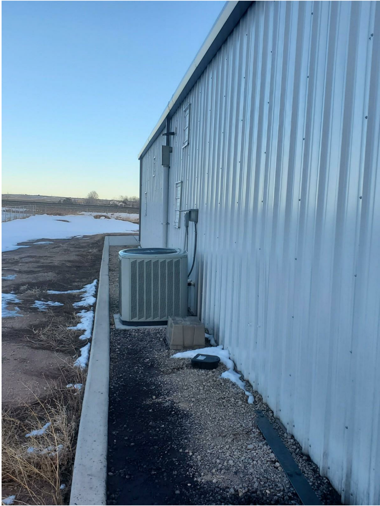
NW CORNER LOOKING EAST
